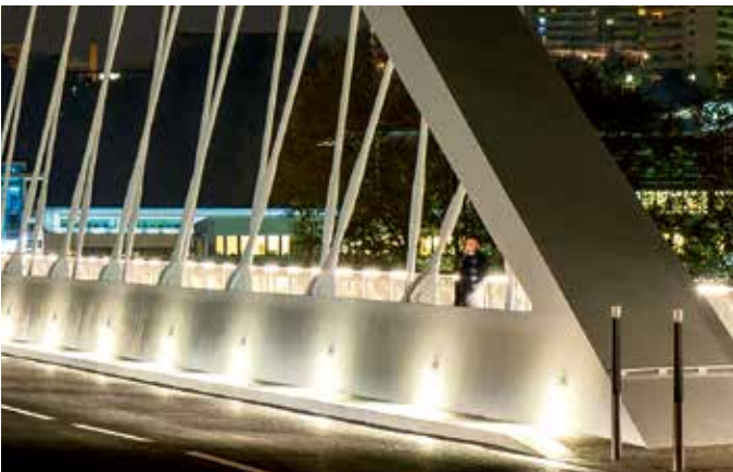
1 Lighting Control — Pont Schuman, Lyons The plan involved the placement of the light sources at just 28 centimeters (11 inches) above the ground. With a specially developed lens shape, ewo brings non-dazzling light to the street that meets the EN 13201 standard, even from this low height. ➤ pp. 66–67
