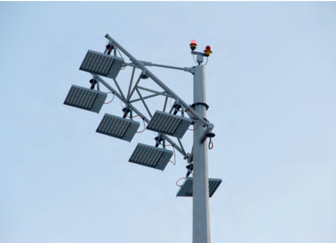
The LED floodlight is mounted onto the existing holder.
