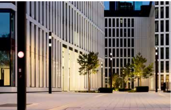
4 Additional Functions — St Martin Tower, Frankfurt The steles illuminate toward two sides and additionally integrate elements of the intercom installation, a traffic light system, video cameras, and tank ventilation. ➤ pp. 41–43
