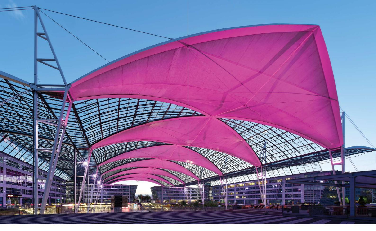
Flexible light distribution by means of a dynamic control system that allows the activation of a range of programmed scenes as required
